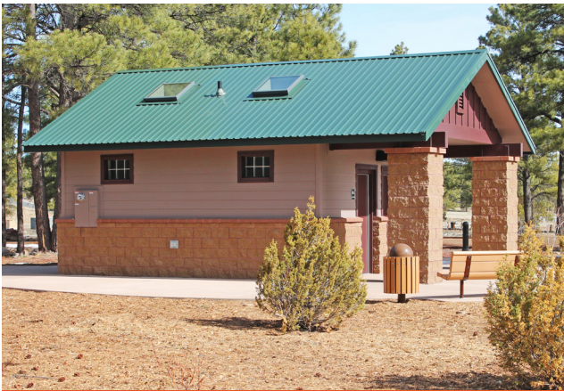
The Cataract Lake County Park renovation included replacing the existing park amenities ranging from ramadas to bathroom facilities.
