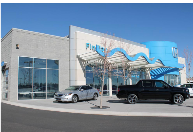
The Findlay Honda is a structural masonry facility built using concrete slab-on-grade construction.
