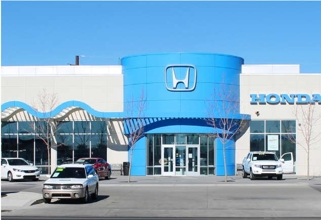
The Findlay Honda features a 3,500SF showroom, a 4-bay quick lube center, a 5,700SF, and 10-bay service center garage.
