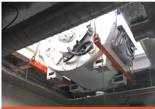
Project included construction of a new roof opening for use during this MRI installation and for future equipment upgrades.
