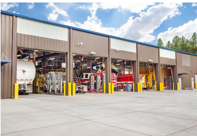
The Public Works Yard hosts the City's new vehicle maintenance building, streets building, parks building, vehicle fueling facility, cold weather vehicle wash building, and administration building.
