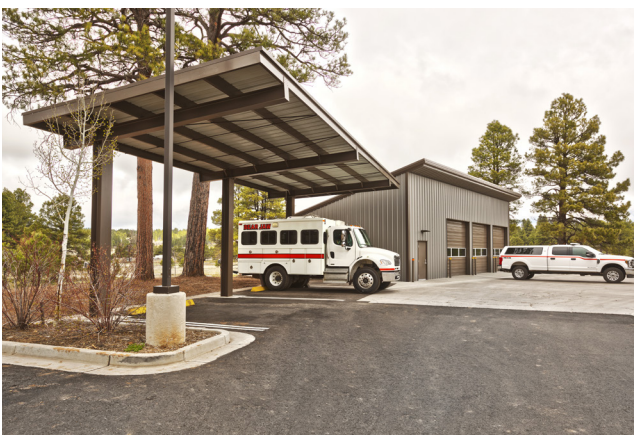
New Bear Jaw Wildfire Crew quarters offer a much needed upgrade for staging and gear maintenance.
