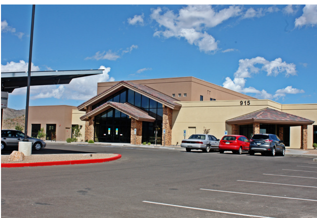
Expanded parking includes photovoltaic energy integrated into the shade structures.
