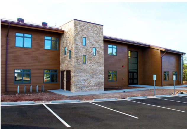
During preconstruction, it was determined that re-siting the building to an existing brownfield would produce significant savings for the National Park Service and would garner additional points in the LEED Certification process. This new site also enabled a re-orientation of the planned structure to maximize solar benefits.
