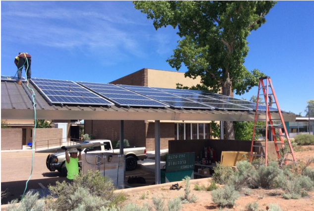
Loven Contracting constructed a shade structure with a photovoltaic array.
