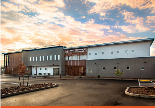
Loven Contracting worked with Sunset Community Health Center to build their new clinic building in Yuma, AZ.
