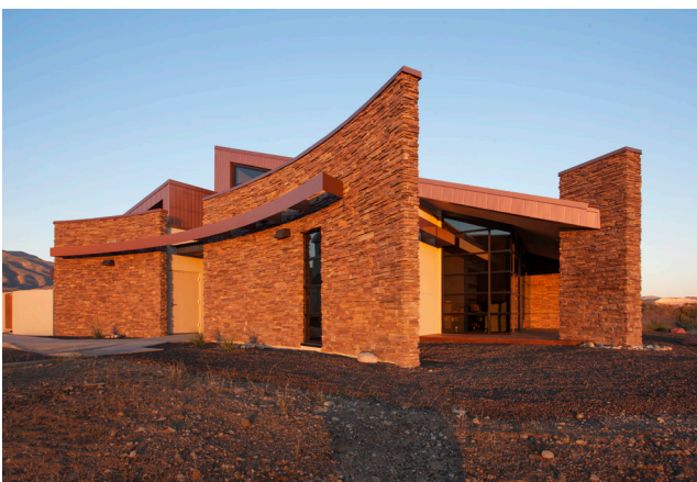
The Hospice House hosts a meditation room, physician consultation room, a nurse's station, and office.
