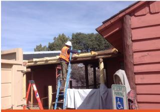
Loven Contracting self-performed intricate carpentry work to replicate the historic textures of the original logs/vigas via modified modern tools for efficiency and accuracy.
