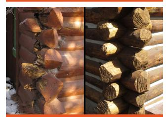
Southeast log crown before and after the preservation process illustrating preserved logs, board and batten wood siding, wood shakes, excavated stone foundation, and the addition of a fully reversible copper gutter and downspout. Great care was taken by our team's carpenters to accurately select all logs for repairs and to duplicate their historic shape and tool marks.
