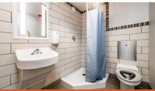
The behavioral health facility is equipped with tamper-proof MEP components and ligature-resistant features throughout. Examples in patient restrooms include recessed back-lit and impact resistant mirrors, ligature-resistant door handles, soap dispensers, sink, and recessed hands-free flushometers.
