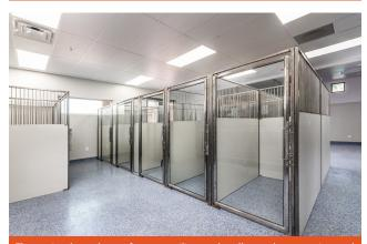
The canine kennel area features ceiling and wall sound attenuation and half-height PVC isolation panels on the kennels to reduce animal stress and noise. Non-absorbent epoxy flooring is durable and easy to sanitize.
