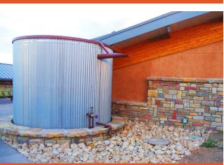
Sustainability features included upgrades to rain-water harvesting systems and the installation of a new catchment system and water storage tank, as well as a new photovoltaic system for solar integration.
