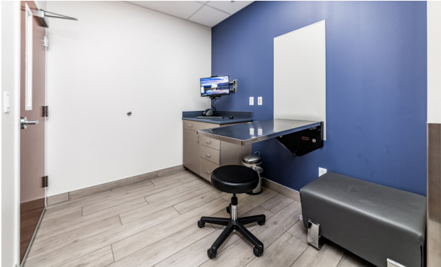
Private exam rooms are equipped with a fold down table and FRP wall panel for flexibility of use, and the porcelain plank floor tiles are aesthetically pleasing and resilient. In addition to the standard exam rooms, space inventory includes specialty feline exam, outdoor exam, and euthanasia comfort rooms.
