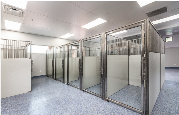
The canine kennel area features ceiling and wall sound attenuation and half-height PVC isolation panels on the kennels to reduce animal stress and noise. Non-absorbent epoxy flooring is durable and easy to sanitize.
