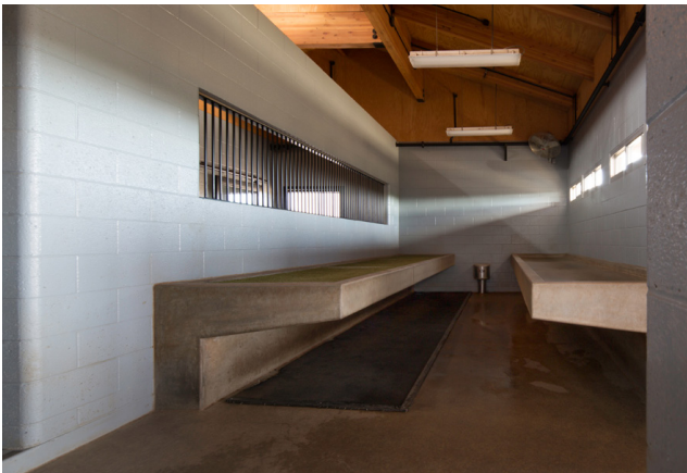
The cast-in-place concrete kennel beds incorporate heating systems and provide warm or cool bed options for the dogs.
