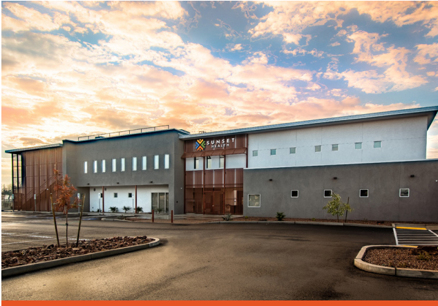
Loven Contracting worked with Sunset Community Health Center to build their new clinic building in Yuma, AZ.
