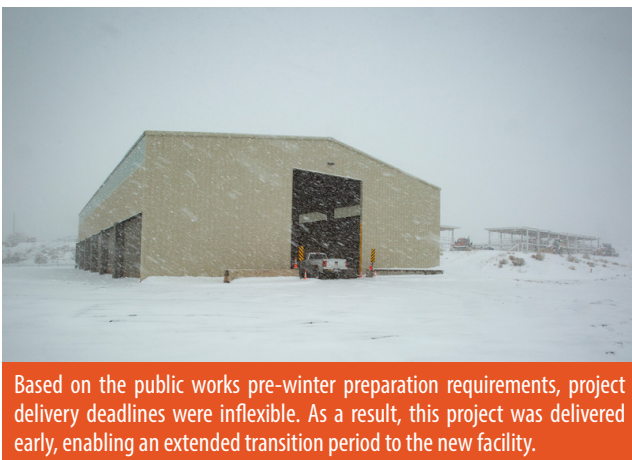
Cinder barn openings were calculated based on loading equipment specifications, reducing the number of required maneuvers by equipment operators.
