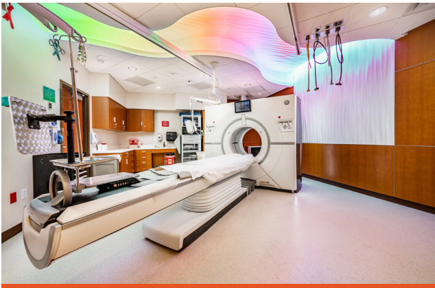
This Design + Build project included a programmable LED "river" as a part of improving the overall quality of patient experience.
