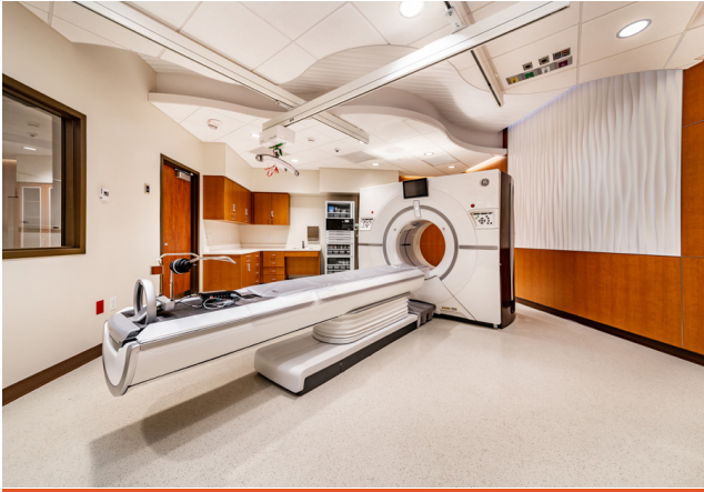
This tenant improvement included a new layout, MEP / med gas upgrades, and new imaging equipment installation.
